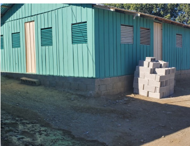
Bricks for the bathrooms walls
